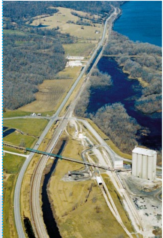
Holcim, Inc., near Clarksville, Missouri, taps rich resources to manufacture cement (right). In partnership with the Little Dixie Highway, a new Interpretive Center will explain the manufacturing process (opposite).
