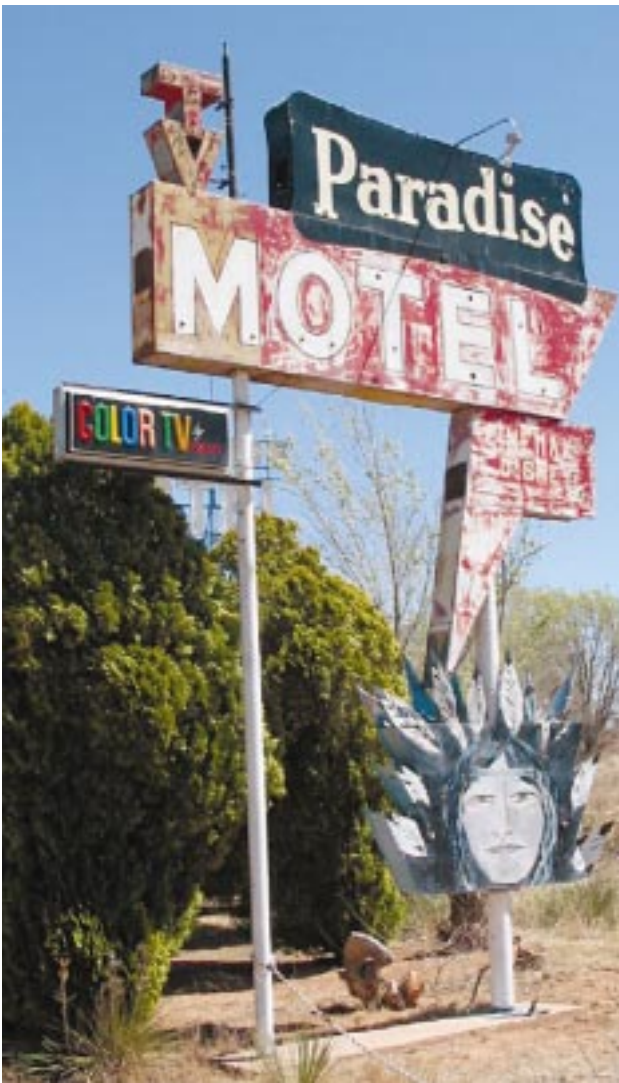
Paradise Motel, Tucumcari, NM, before restoration (left). The Paradise Motel after restoration in December 2002 (above).
