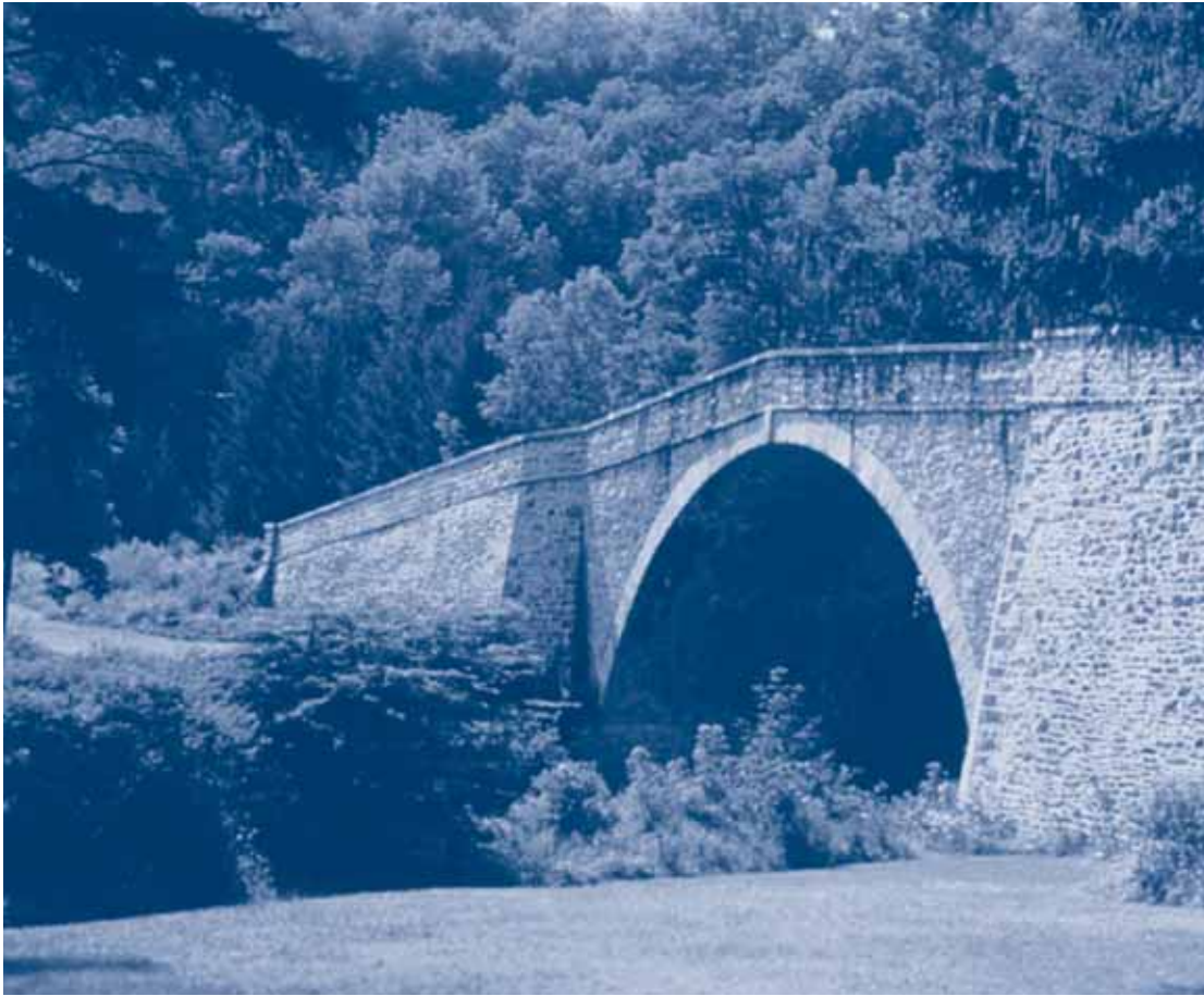
The best-known and most magnificent National Road stone bridge in Maryland is the bridge at Little Crossings, called the Casselman River Bridge. Built on a tributary of the Youghiogheny River in 1813, this structure was the longest span of any stone bridge in the nation at the time of its construction. © 2000. Lardner/Klein Landscape Architects.
