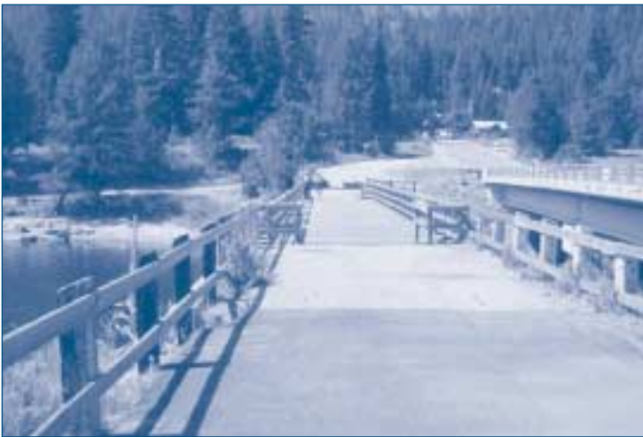
The Tamarack Falls Recreation Area features a handicapped-accessible fishing bridge parallel to the road. Credit: Payette River Scenic Byway Advisory Council
