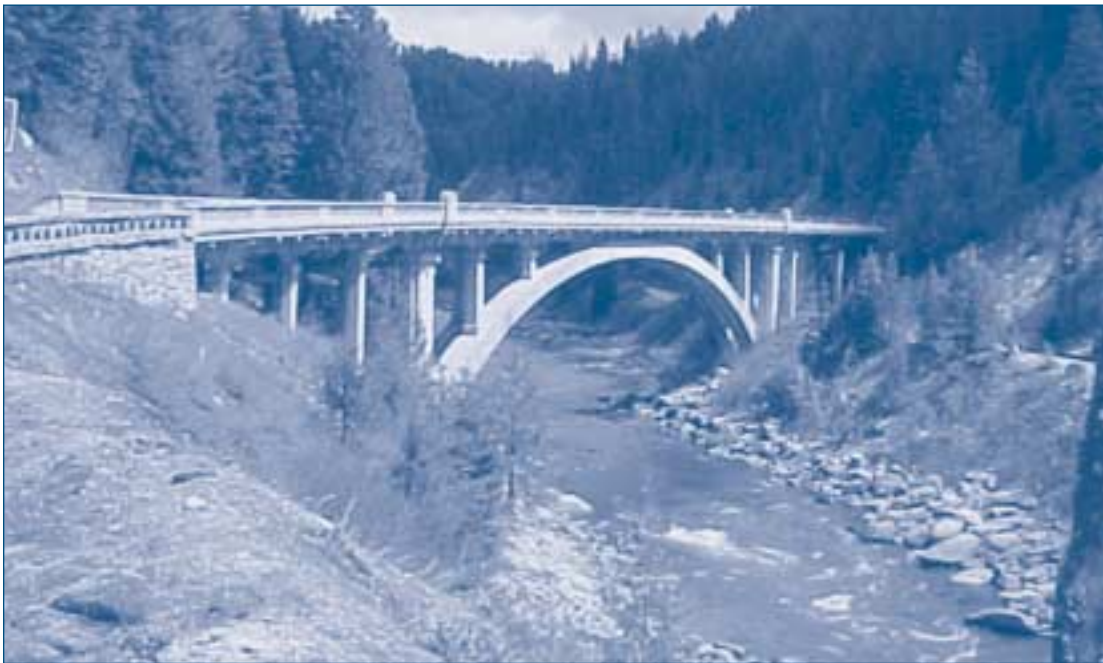
The Rainbow Bridge, built in 1933, is listed on the National Register of Historic Places for its engineering design. Credit: Marianne Piquet
