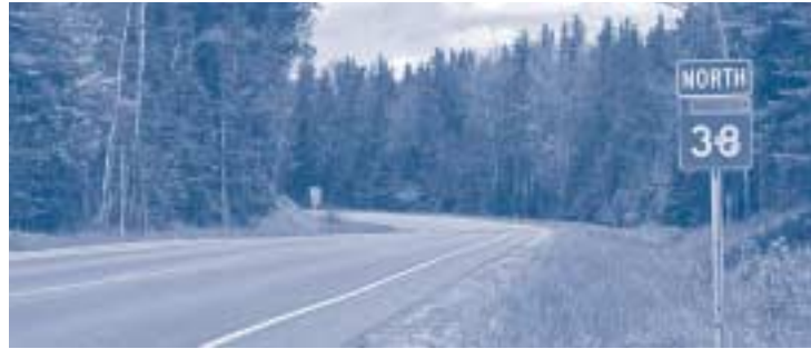
AASHTO awarded the Minnesota Department of Transportation for its extraordinary development and reconstruction of Minnesota Highway 38, "Edge of the Wilderness National Scenic Byway." Photo Credit: Mn/DOT, Neil Kveberg
