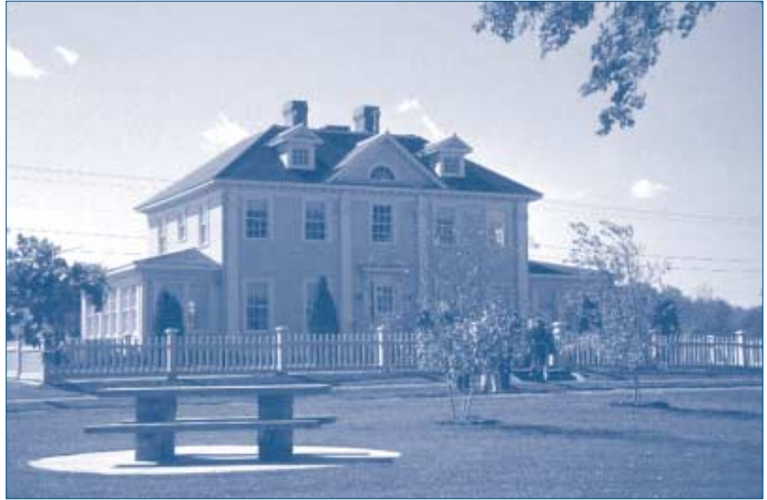
The Federal Highway Administration, Minneapolis Park and Recreation Board, the Minnesota legislature, the Longfellow Restoration Group and the Longfellow Neighborhood worked together with the Grand Round National Scenic Byway to restore the historic Longfellow House. It now serves as the byway’s gateway information center.
